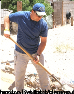
Excavating a site for a foundation. Photo by: [Name]
